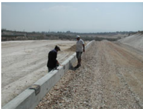
Casting a concrete beam
