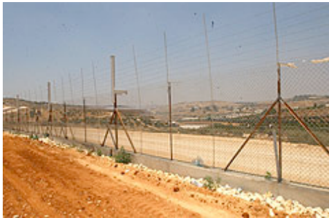
Intrusion detection fence
