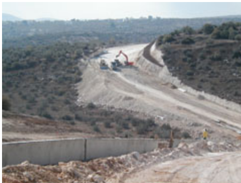
Paving a road in the Salem Elkana area - first stage
