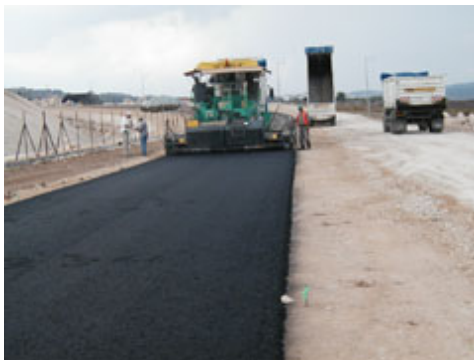
Paving a road in the Salem Elkana area
