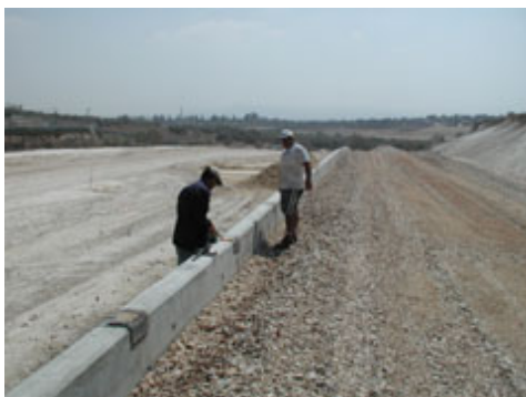
Casting a concrete beam
