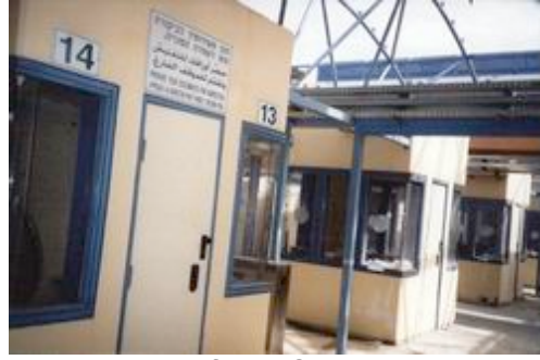
Inside view of the Crossing under construction.
