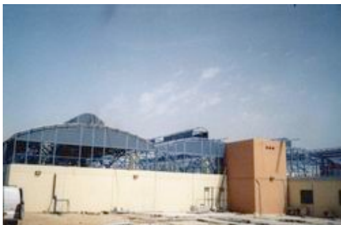
External view of the Crossings under construction
