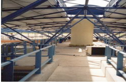
Inside view of the Crossing under construction.
